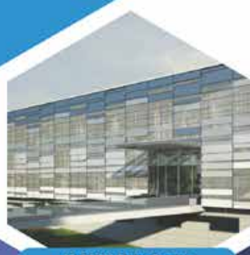
IS BANK Data Center
