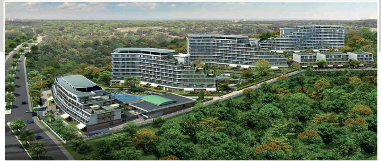
Kurtköy Housing Project, İstanbul
